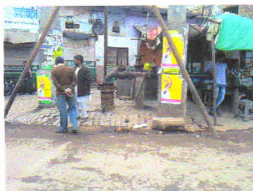
Picture 5.2: Ground water pumping system at Jaunpur (near ShahiQila)
