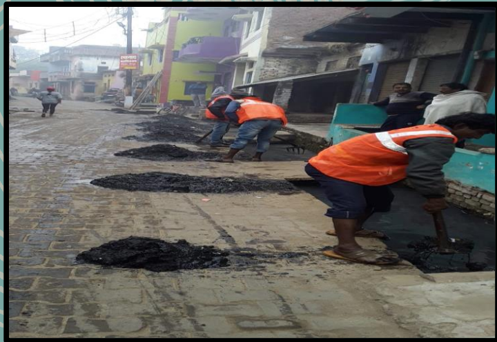
Drain cleaning on daily basis
