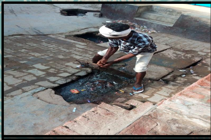
Drain cleaning on daily basis
