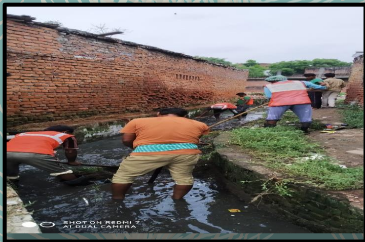
Drain cleaning on daily basis
