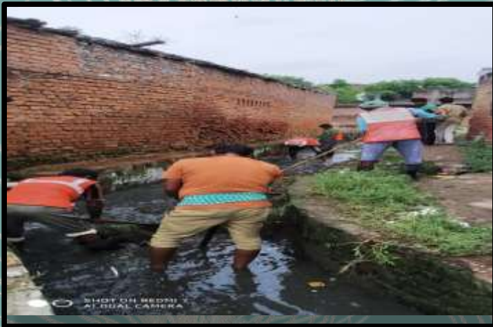
Drain cleaning on daily basis
