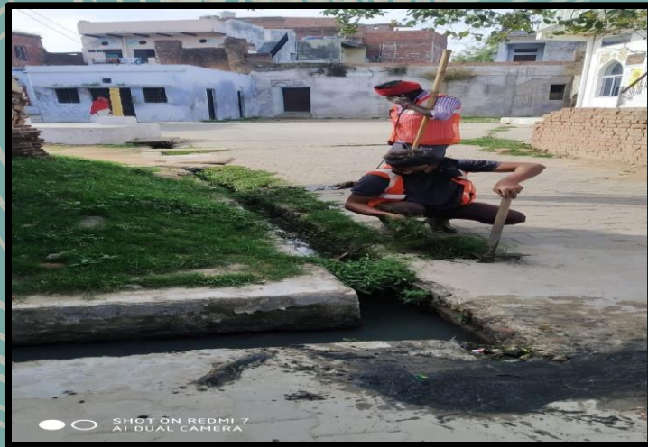
Drain cleaning on daily basis
