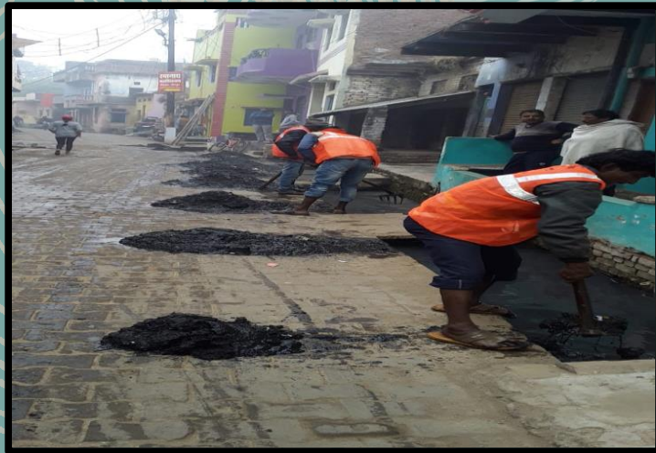
Drain cleaning on daily basis
