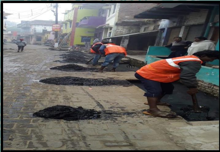
Drain cleaning on daily basis
