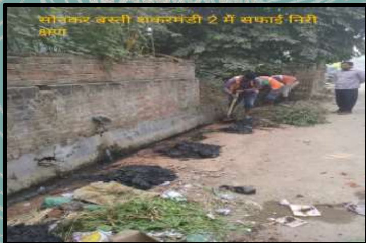
Drain cleaning on daily basis
