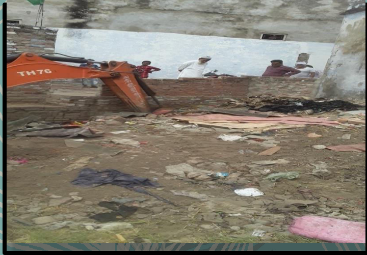
Drain cleaning on daily basis
