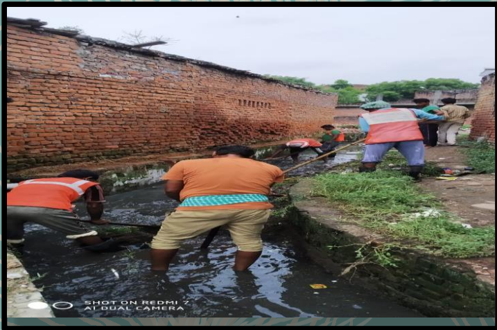
Drain cleaning on daily basis
