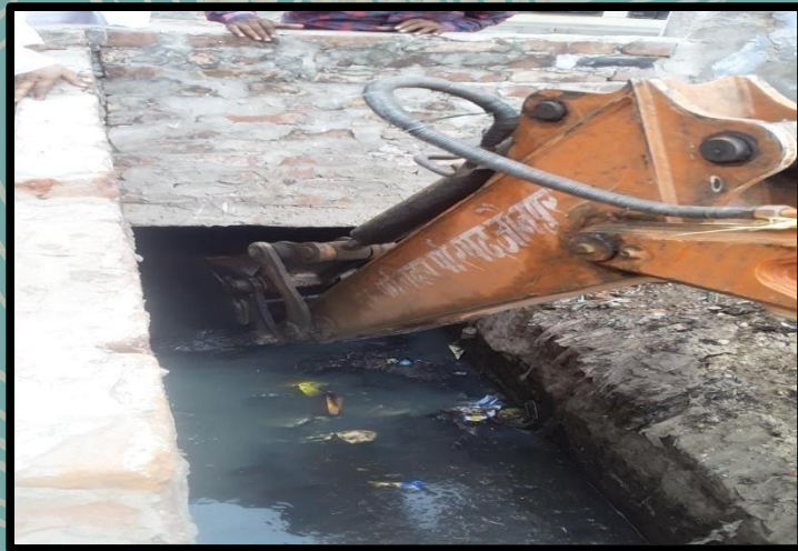
Drain cleaning on daily basis
