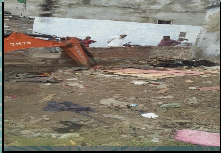
Drain cleaning on daily basis
