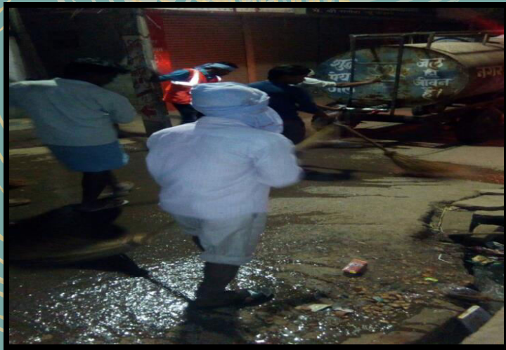
Drain cleaning on daily basis
