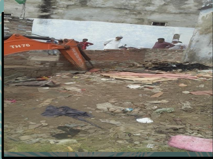
Drain cleaning on daily basis
