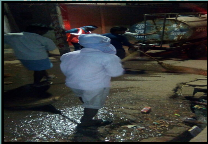
Drain cleaning on daily basis
